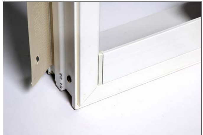
Figure 4: Set new liner in place.
