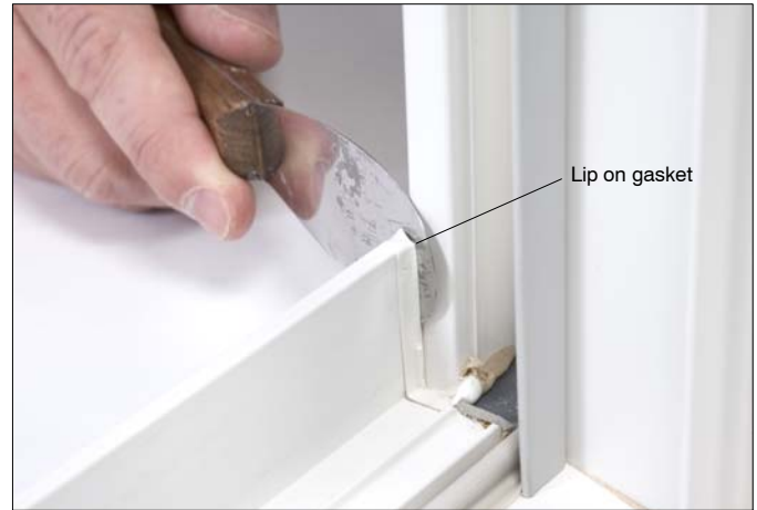
Figure 6: Use putty knife to make sure lip on gasket surrounds jamb.
