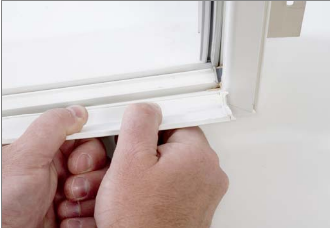
Figure 1: Remove existing sill liner.
