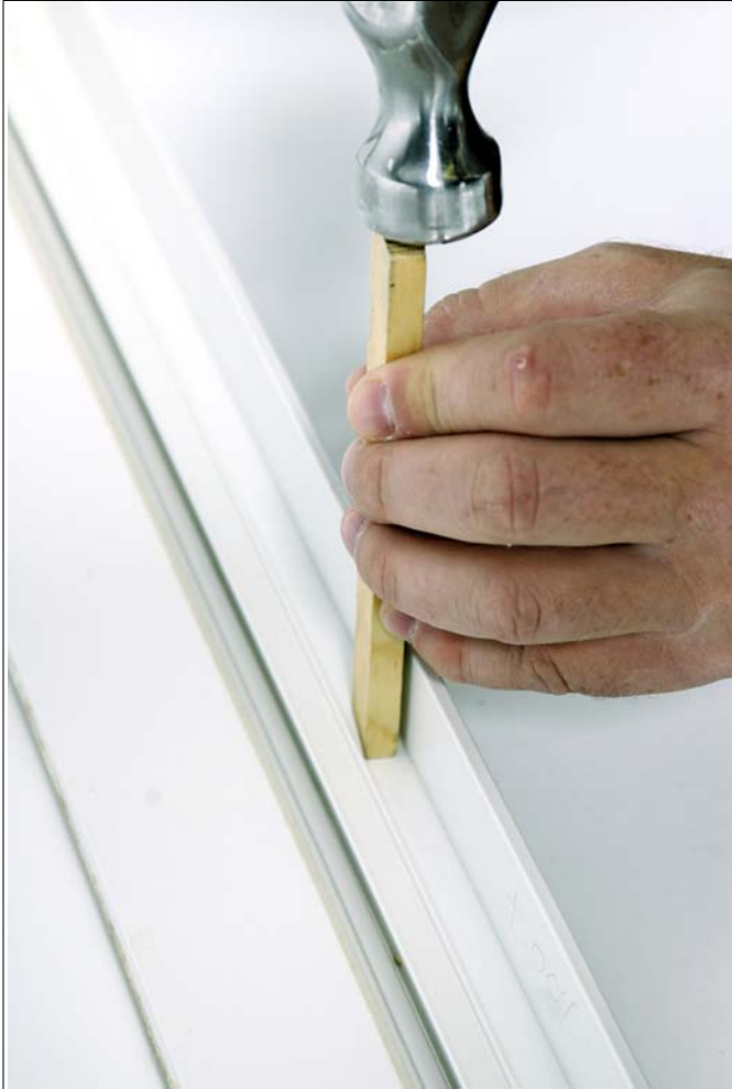
Figure 5: Seat the sill liner in the sill kerf.
