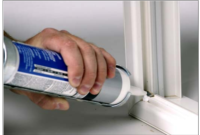
Figure 3: Add sealant to kerf corners.
