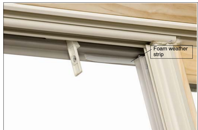
Figure 4: Slide head jamb bracket out of the way of sash.
