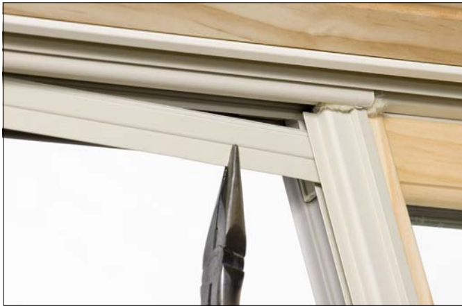
Figure 1: Remove head jamb screen stop.
