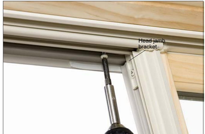
Figure 3: Remove fasteners from head jamb bracket.
