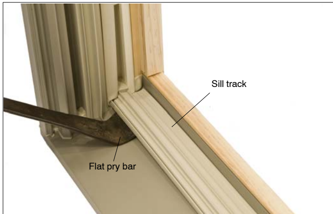
Figure 1: Removing existing sill track.
