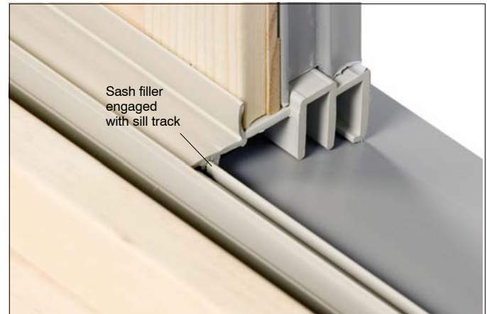
Figure 8: Replace stationary sash.
