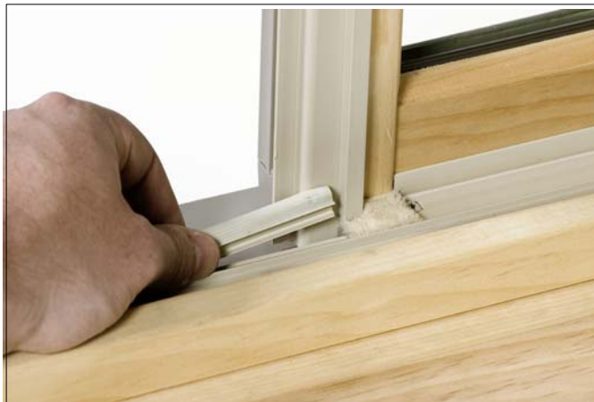
Figure 2: Remove all weather strip.
